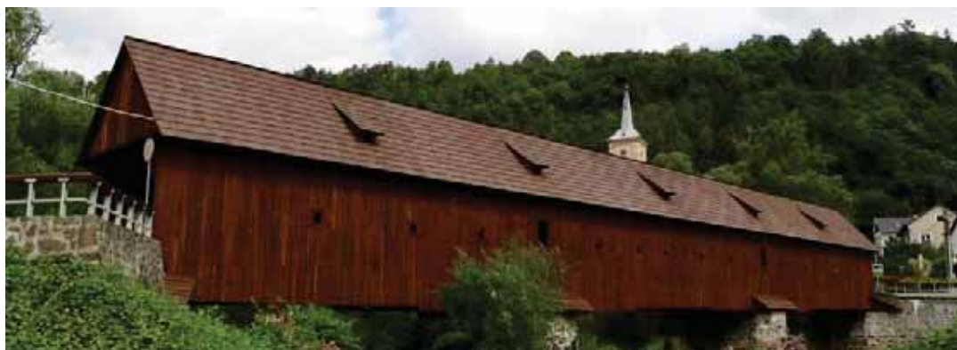
obr. 12: Most Radošov - po obnove
